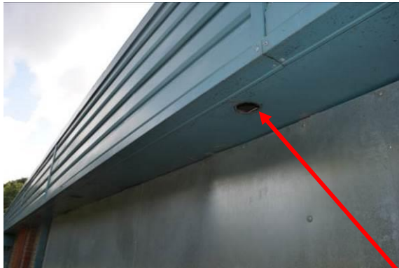
Figs. 17 & 18 External gaps cont'd (arrowed)
