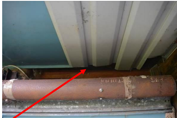
Figs. 17 & 18 External gaps cont'd (arrowed)
