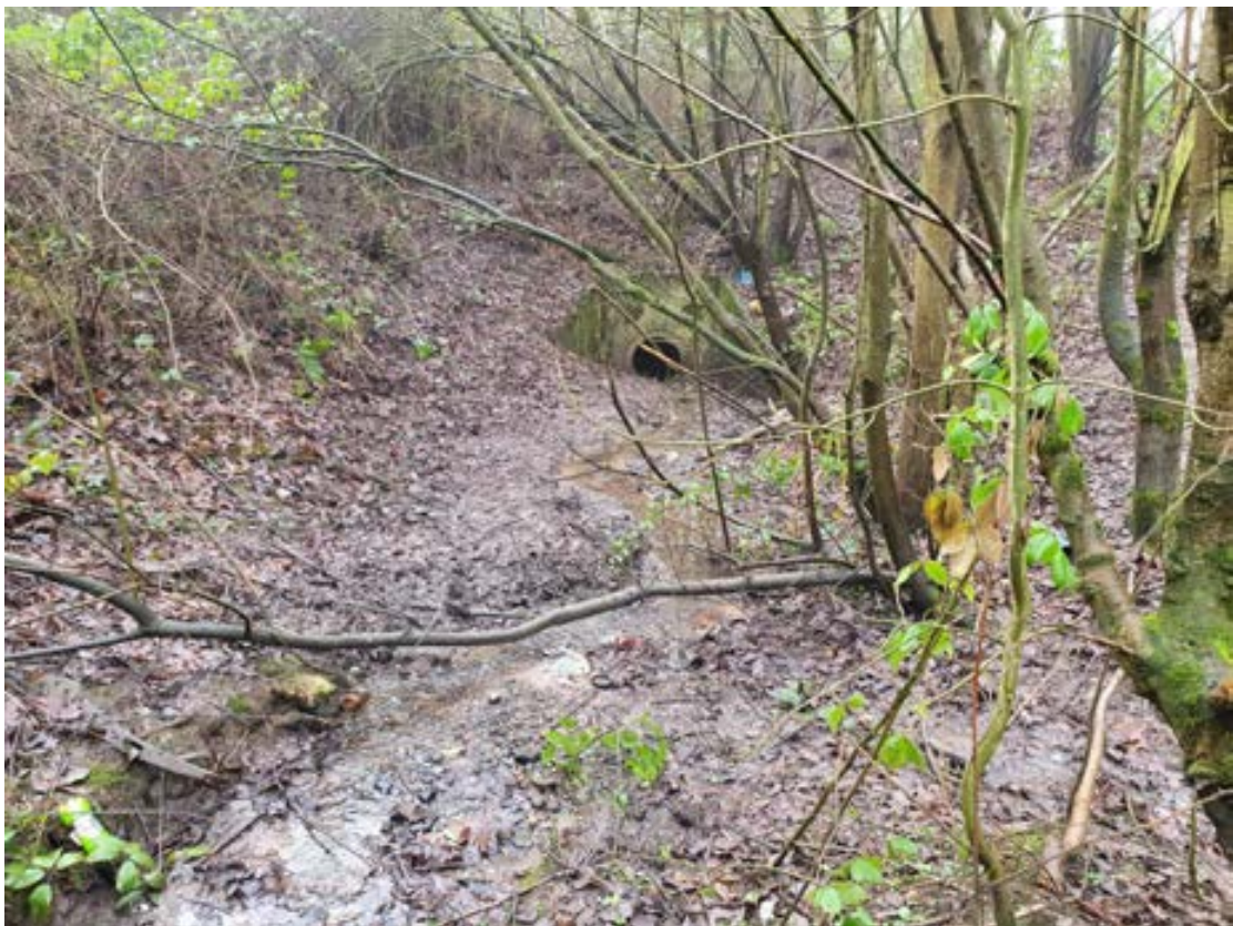
Photograph 10: Inflow pipe seen at the start of the watercourse on site.
