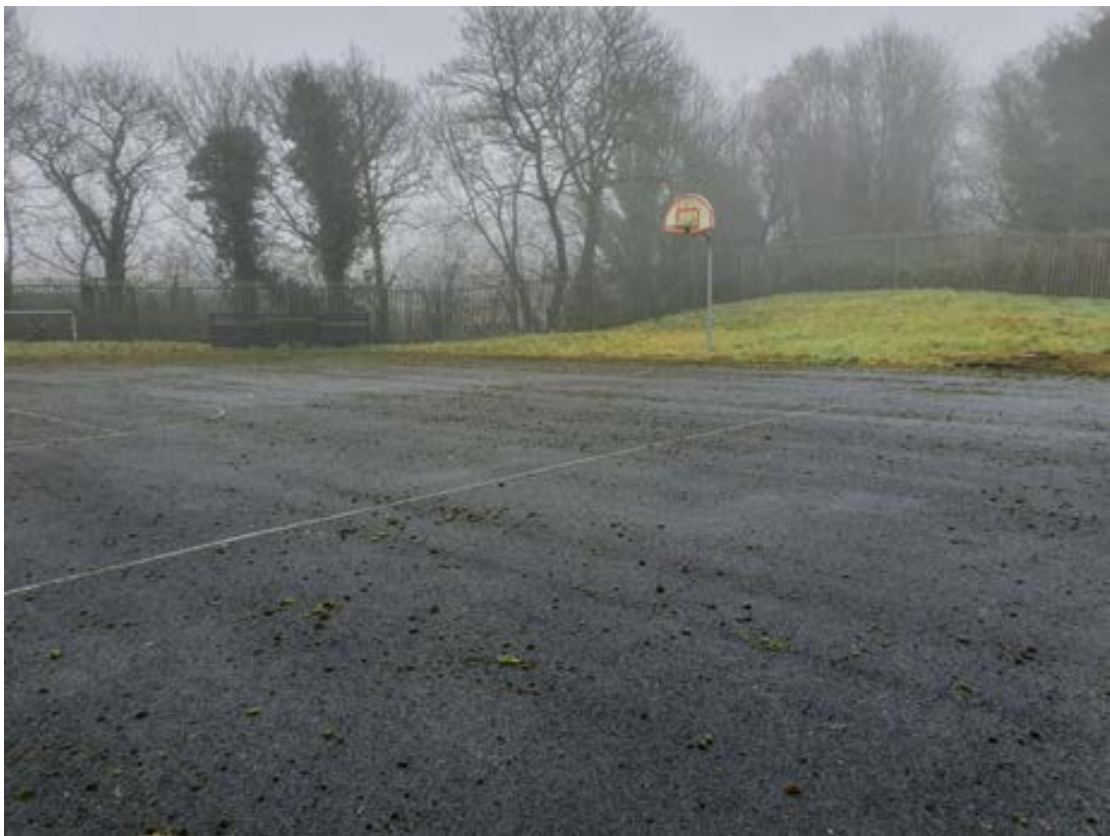
Photograph 4: Hardstanding used for sports activities and palisade fence surrounding the school grounds.
