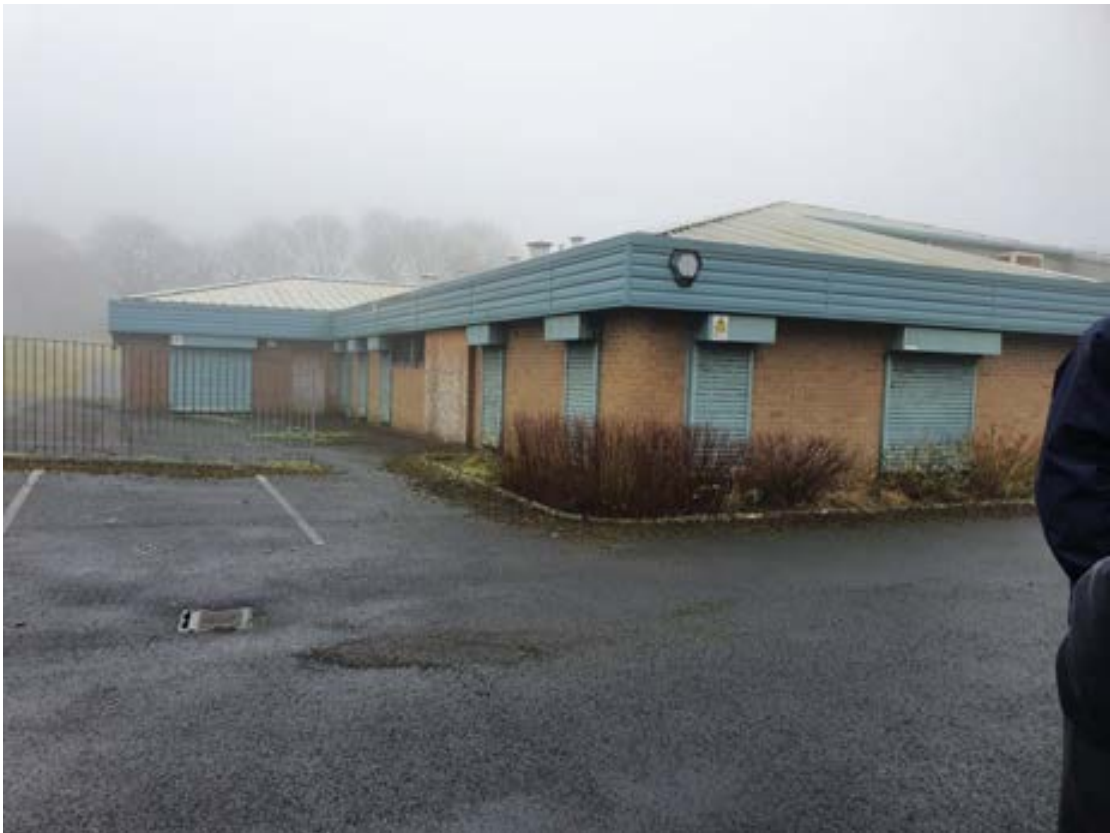
Photograph 2: Unoccupied Hope High School, comprising brick and corrugated steel roof.
