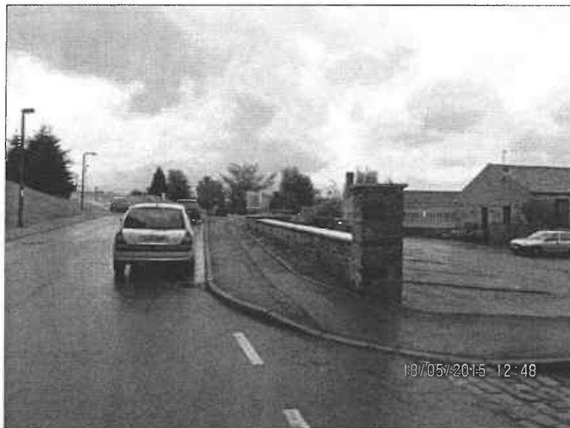
The existing wall fronting Guy Street
