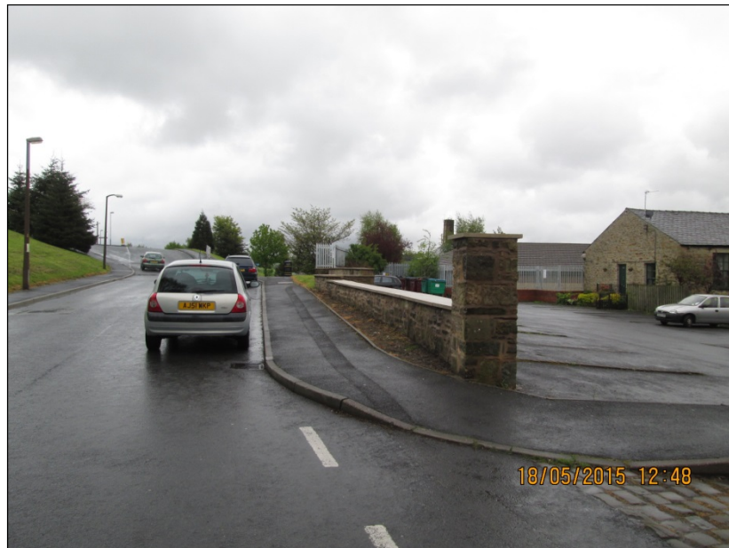
The existing wall fronting Guy Street
