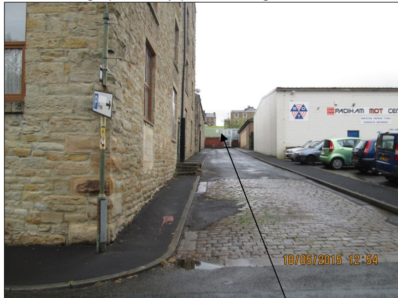
Clitheroe Street – fencing and gate
