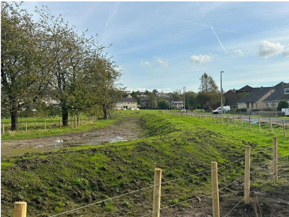
Figure 3: Completed bund (looking south down Lentworth Drive)
