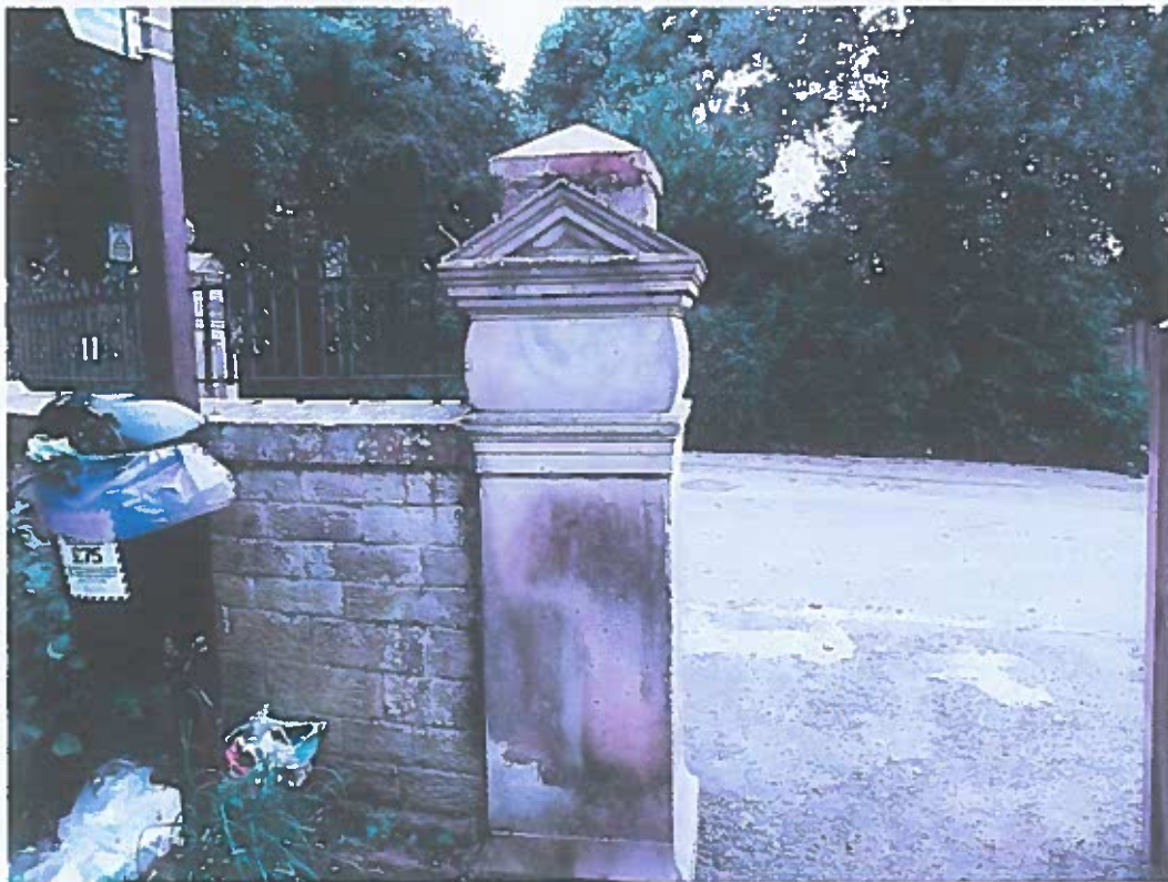
Photo of footpath sign at Plantation Road / Arden Hall entrance (not on line of Definitive Path)
