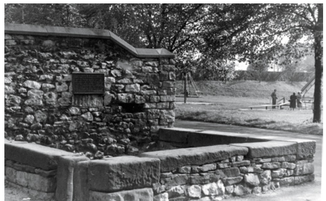
Stock Well, c. 1950. In a recently-wrought change, the higher south-west wall has been lowered to what some maintain was its original Tudor height. All three of Clitheroe's medieval wells have, over the centuries, been subject to many modifications. (Red Rose Collections, ECL20141216014)
