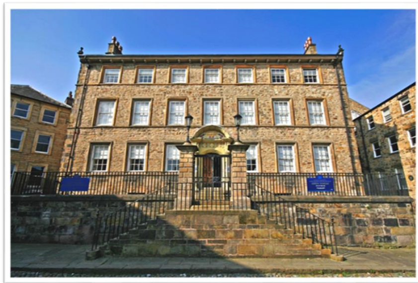
Photo 1. The front of Judges' Lodgings building showing front door and stairs
