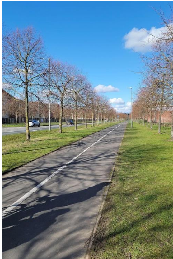
Figure 4-6: Separated Cycle Lane and Footway
