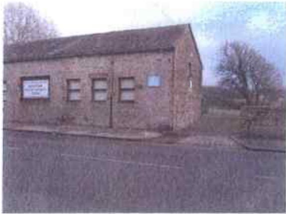
1i. Barton Road Youth and Community Centre (A). Grid ref: 348382,459895
